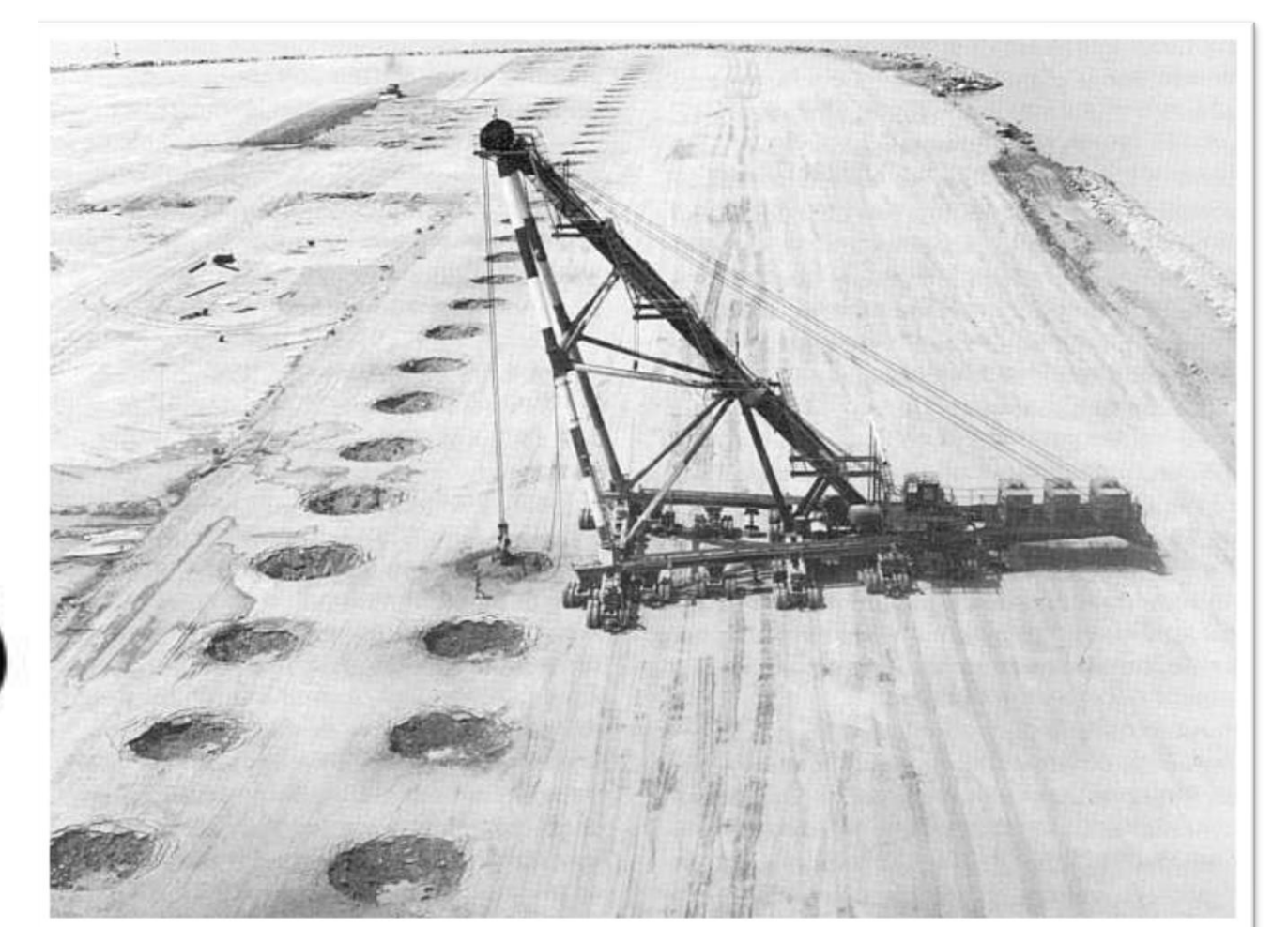
Dynamic compaction techniques were also a contribution by Ménard
